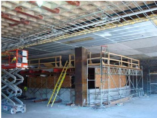
Figure 24: Photo showing the escalator ceiling work.
