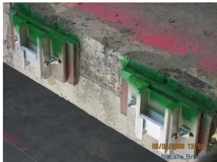
Figure 23: Curtainwall panel's anchors
